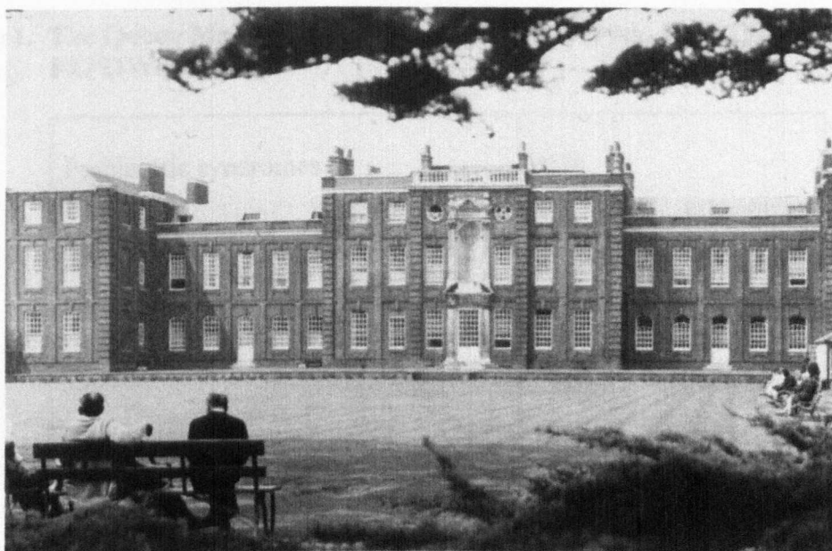
Figure 1. Queen Mary's Hospital, Roehampton in the late 1940s. This military hospital cared for large numbers of ex-Far East POWs in the early post-war years.
