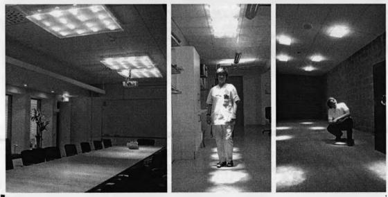
Figure 7.14: Daylight-only luminaire in use.
