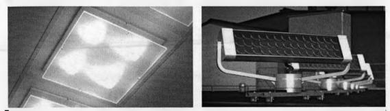
Figure 3.13: Parans system large luminaire for the three generation (left); Parans system collector third generation (right).
