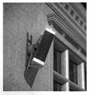
**Figure 4.4:** Light collector influence on building facade, **A**: SCIS collector (left), **B**: Parans 3<sup>rd</sup> generation collector (above)
