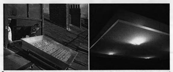
Figure 7.1: Parans solar panel installation in the Uni. Of Livrepool (left); Figure 7.2: Parans 'L1large' luminaire (right).
