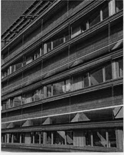
*Figure 3.2:* The anidolic ceiling principle (above); A facade incorporating an anidolic ceiling collector (right).
