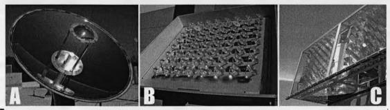
Figure 4.1: Examples for HLS light collectors, A: HSL system, B: Parans system, C: SCIS
