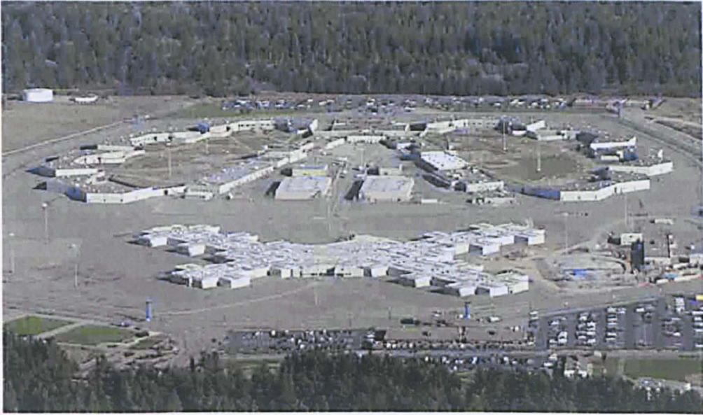
A. Aerial view of Pelican Bay state Prison.**
