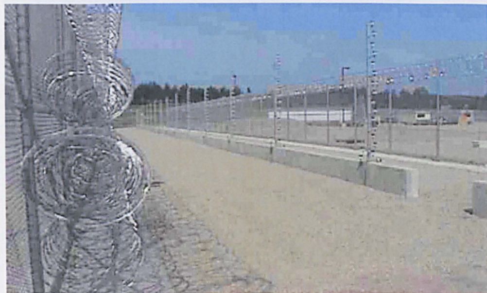
B. Photograph of the perimeter of the supermax facility – two fences with razor wire and sensors between the fences.*
