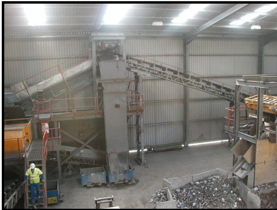
Figure 2-7: A processing plant to produce IBAA (Billingham, Teesside, UK).
