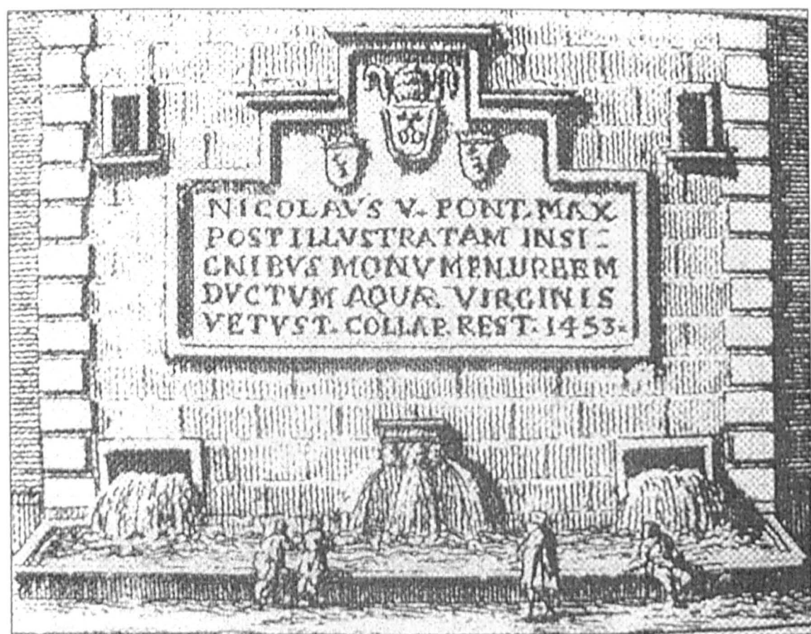
Figure 5-1: The Trevi Fountain, as it appeared in the fifteenth Century, was one of the earliest instances in which theoretical considerations of design and practical requirements of construction were not thought and executed by a single mind. From Manfredo Tafuri, Interpreting the Renaissance : Princes, Cities, Architects , trans. Daniel Sherer (New Haven and London: Yale University Press, 2006).
