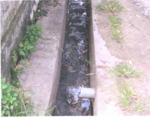
A - a built drain
