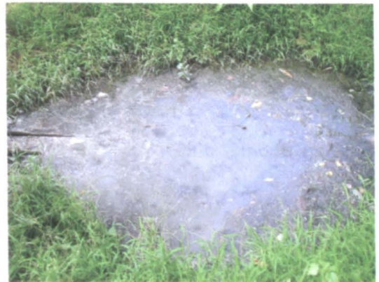
D - an earthen soakage pit
