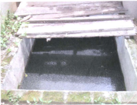
C - a built soakage pit
