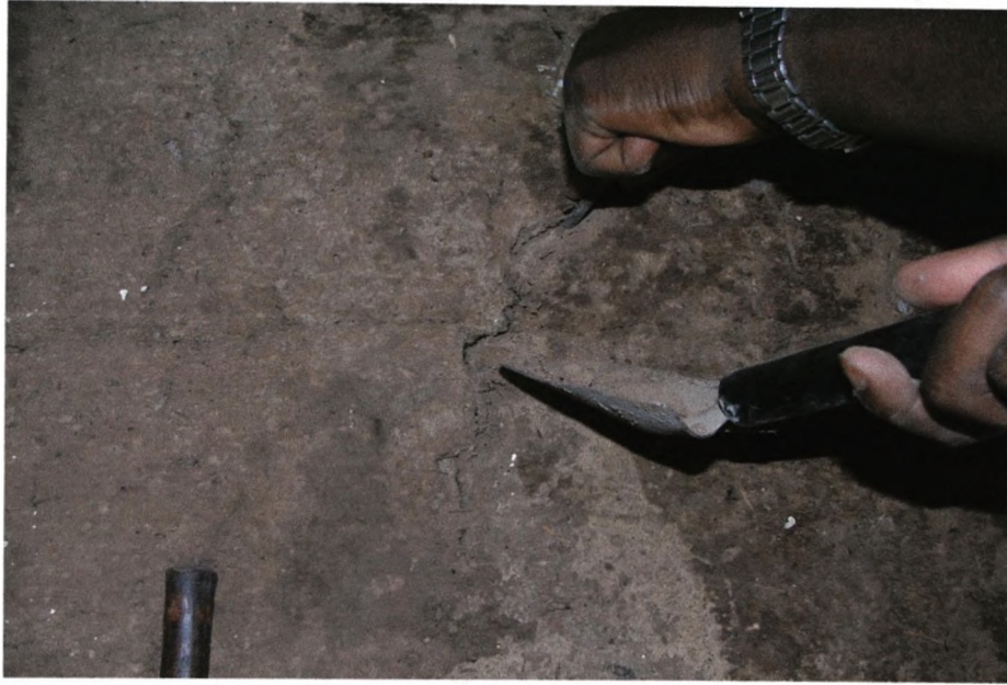
Figure 2.2.2 (a): Sampling of house walls for domestic tick infestations
