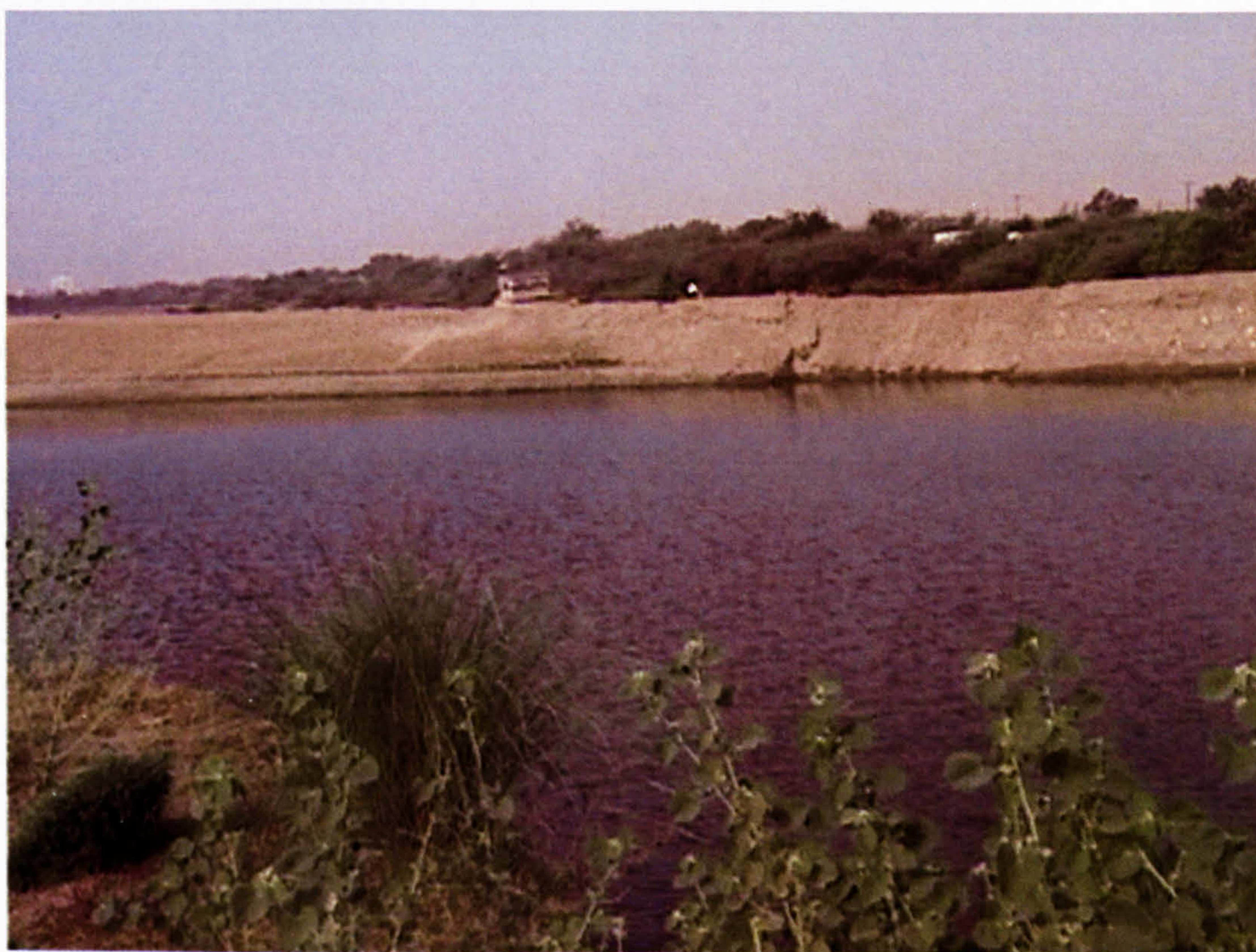
Figure 2.4: Earth dams: They are usually made by local people to store water during the dry season (Feb-July) for agricultural purposes. Al-Megargumm, Jizan region, Saudi Arabia
