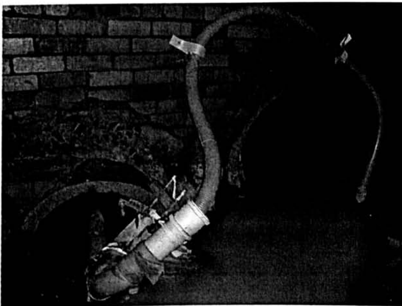
Plate 6.1: Injection of hydrant flow into test section of Forfar 600mm combined sewer
