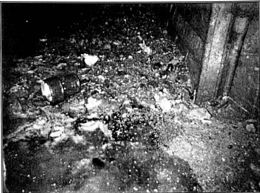
Plate 2.2: Coarse deposits in the Murraygate interceptor sewer
