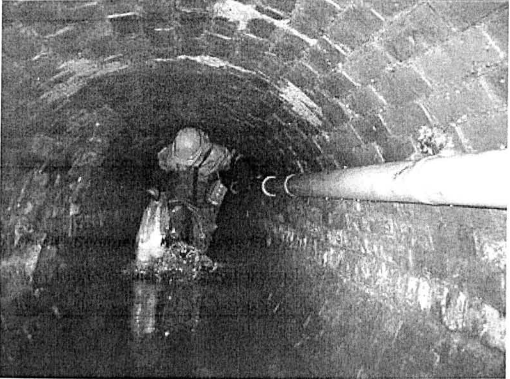
Plate 3.2: Retrieving deposit samples for laboratory analysis
