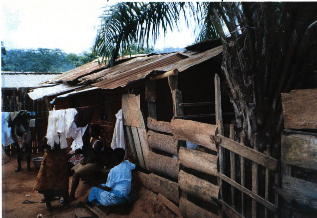
Typical small farm household in Akuapem North: Building is constructed with iron roof, has molten brick walls and plaster
