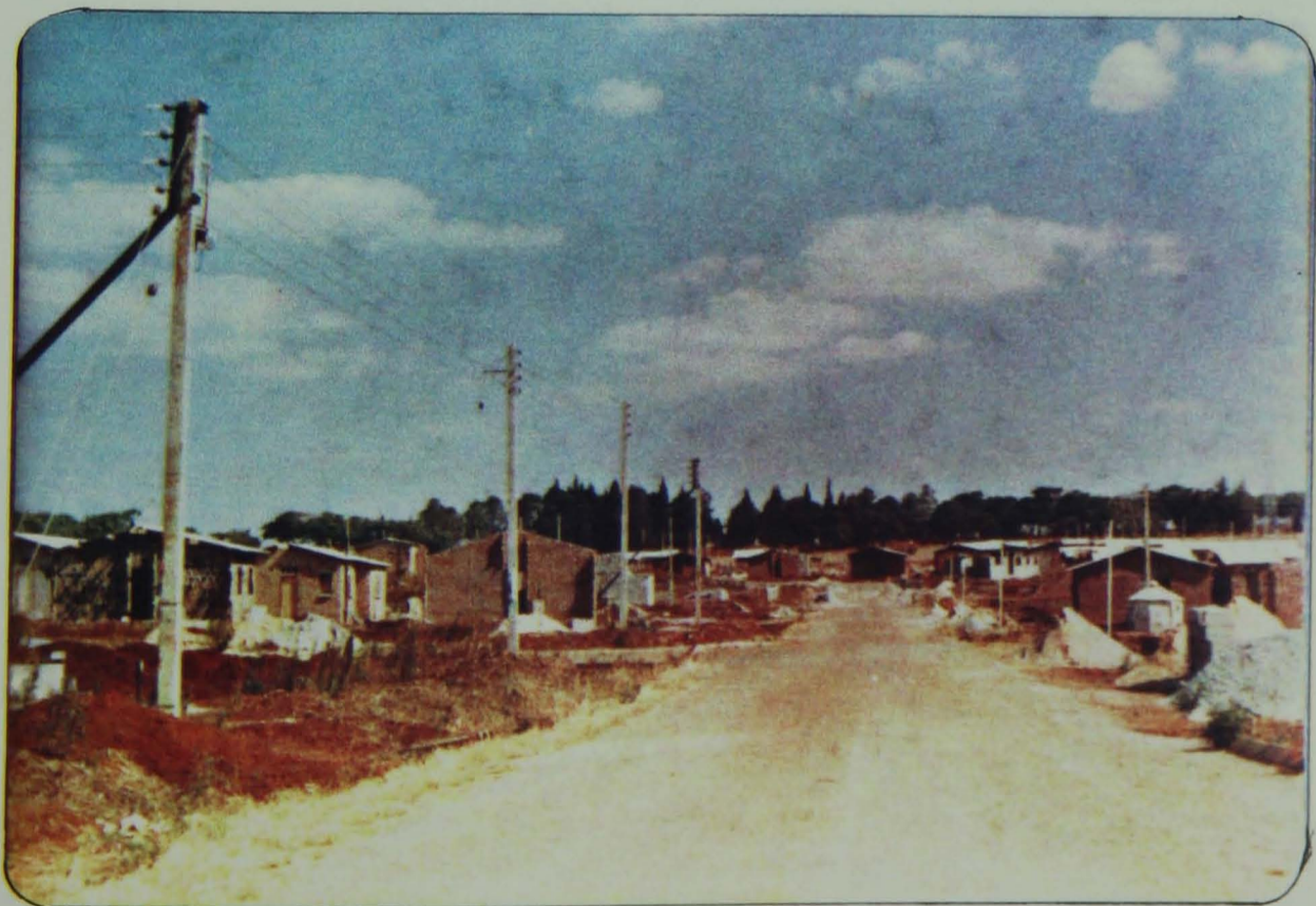
Plate 6.2 - A local distributor road in Hatcliffe. Note the construction taking place and the electrical reticulation already in place. All roads in the newer housing estates are tarred.
