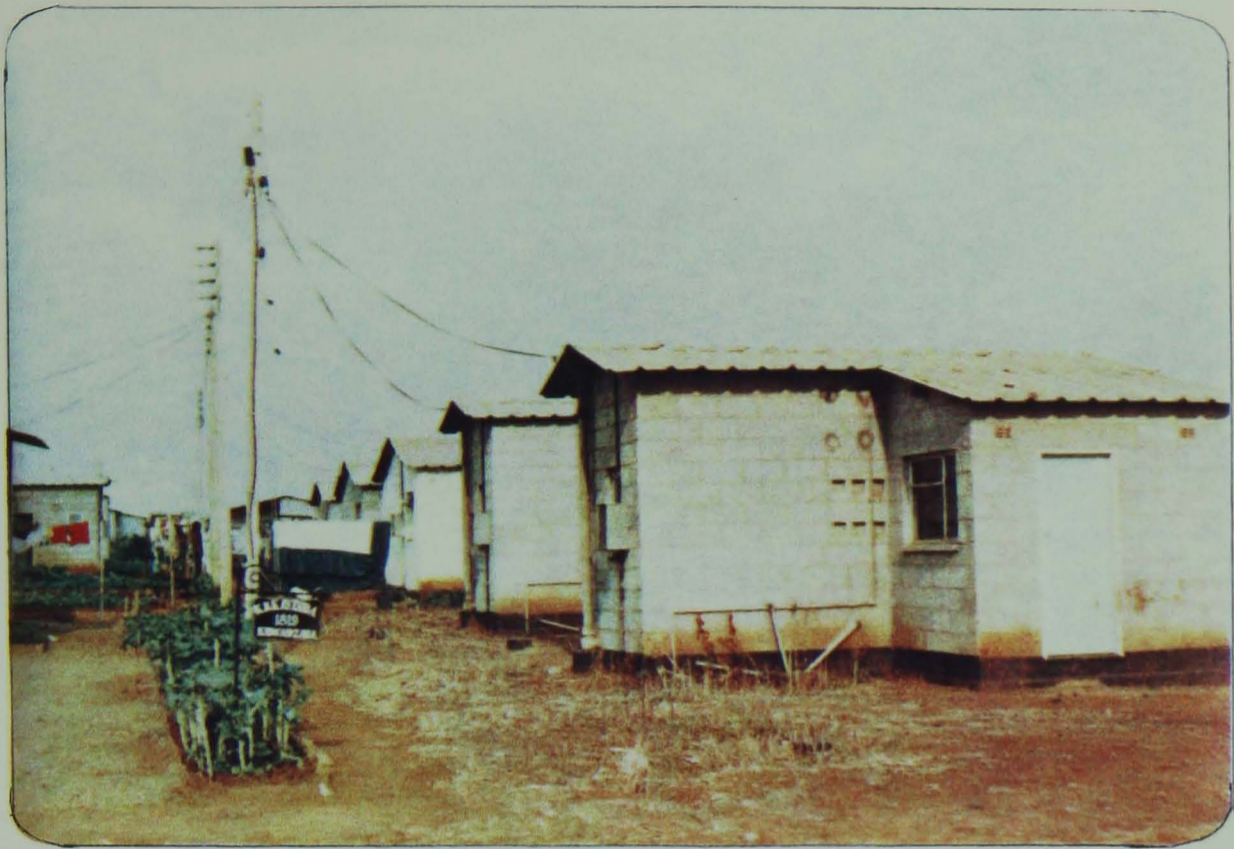
Plate 6.1 - Most services are normally located in servitudes.
