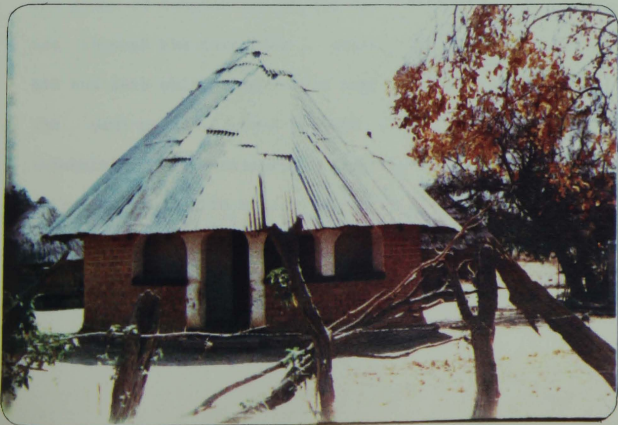
Plate 3.6 - Ingenious use corrugated iron sheets in the roof structure of a rural dwelling. The proud owner nevertheless complained of excessive heat on hot days.
