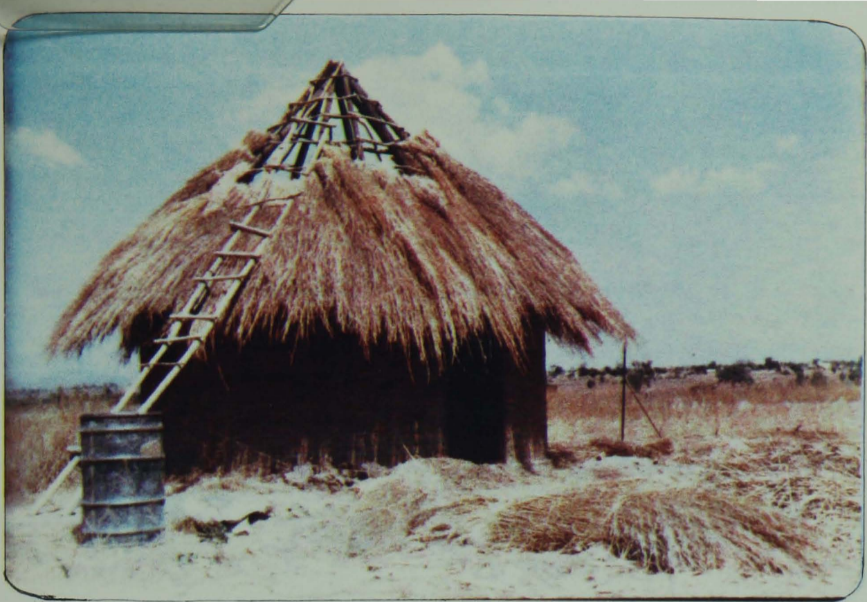
Plate 3.5 - Construction in progress. Note the use of bricks.
