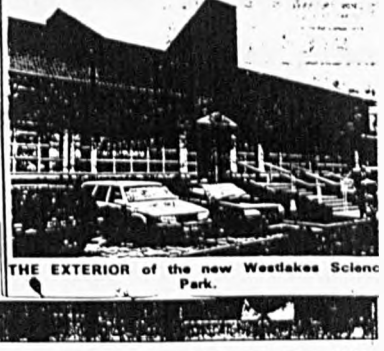
THE EXTERIOR OF THE new Westlakes Science Park.
