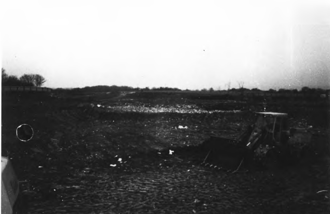
Plate 5. Compaction of Waste at the Tip Face, Etna Landfill Site.
