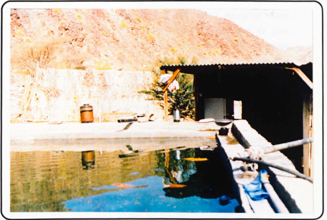
Figure 3.13 Showing cement water basin reservoir in the farm in Wadihaloo village
