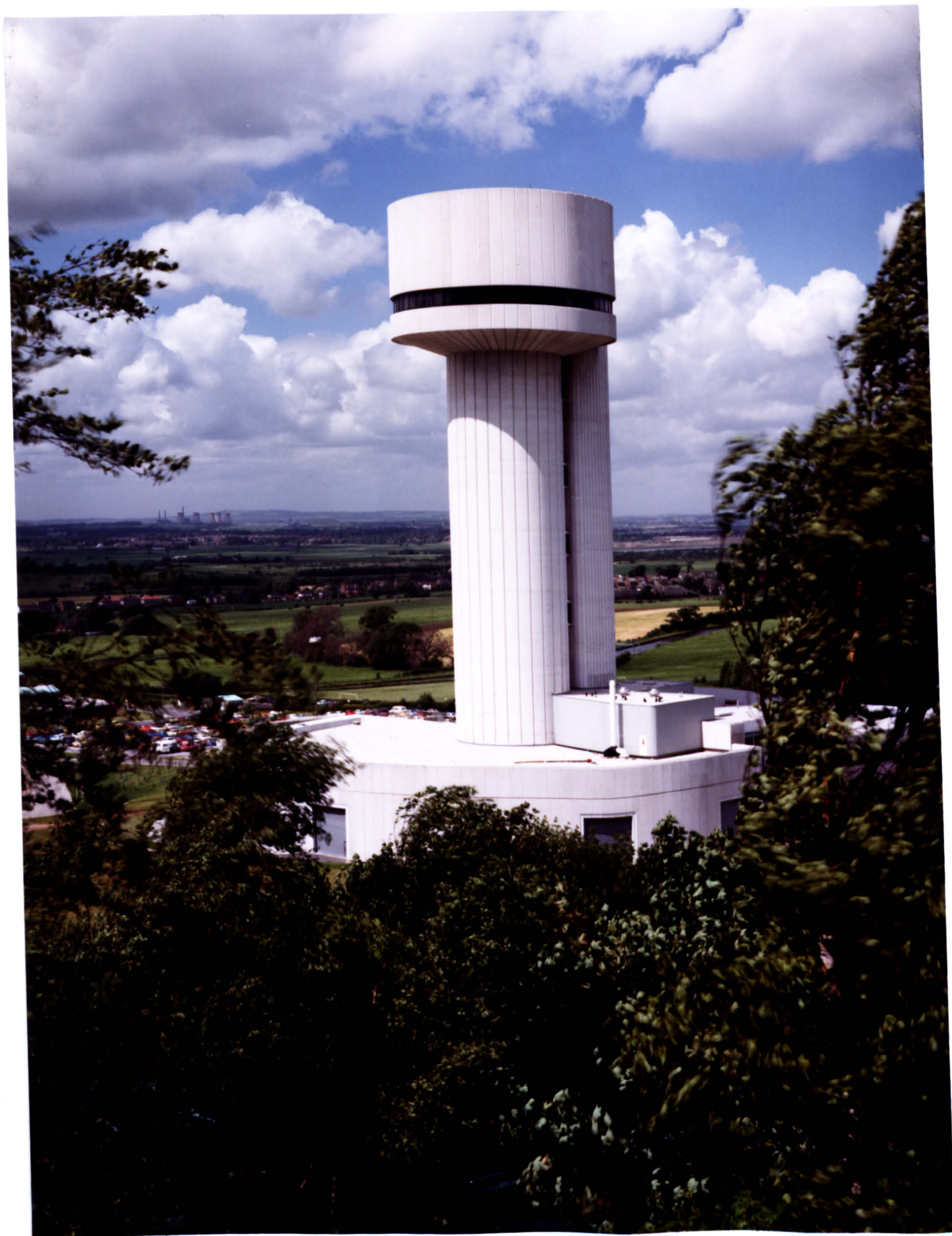
Figure 5.1: The Nuclear Structure Facility (NSF) at Daresbury Laboratory. The 70 m high tower contains a vertical 20 MV tandem accelerator. Ion sources and injector equipment are housed at the top of the tower. The heavy ion beams of the accelerator are employed in the experimental areas inside the hall at the bottom of the building.
