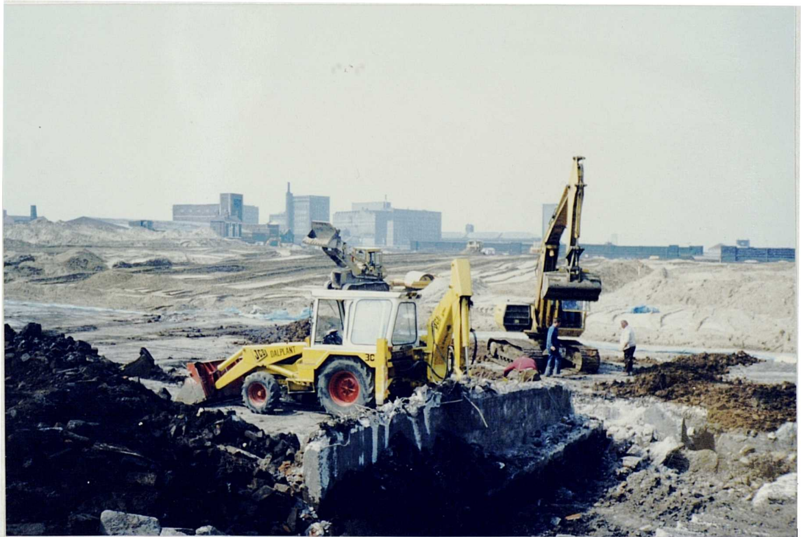
Plate 12. Reclamation in progress at the Tate and Lyle site, May 1987.
