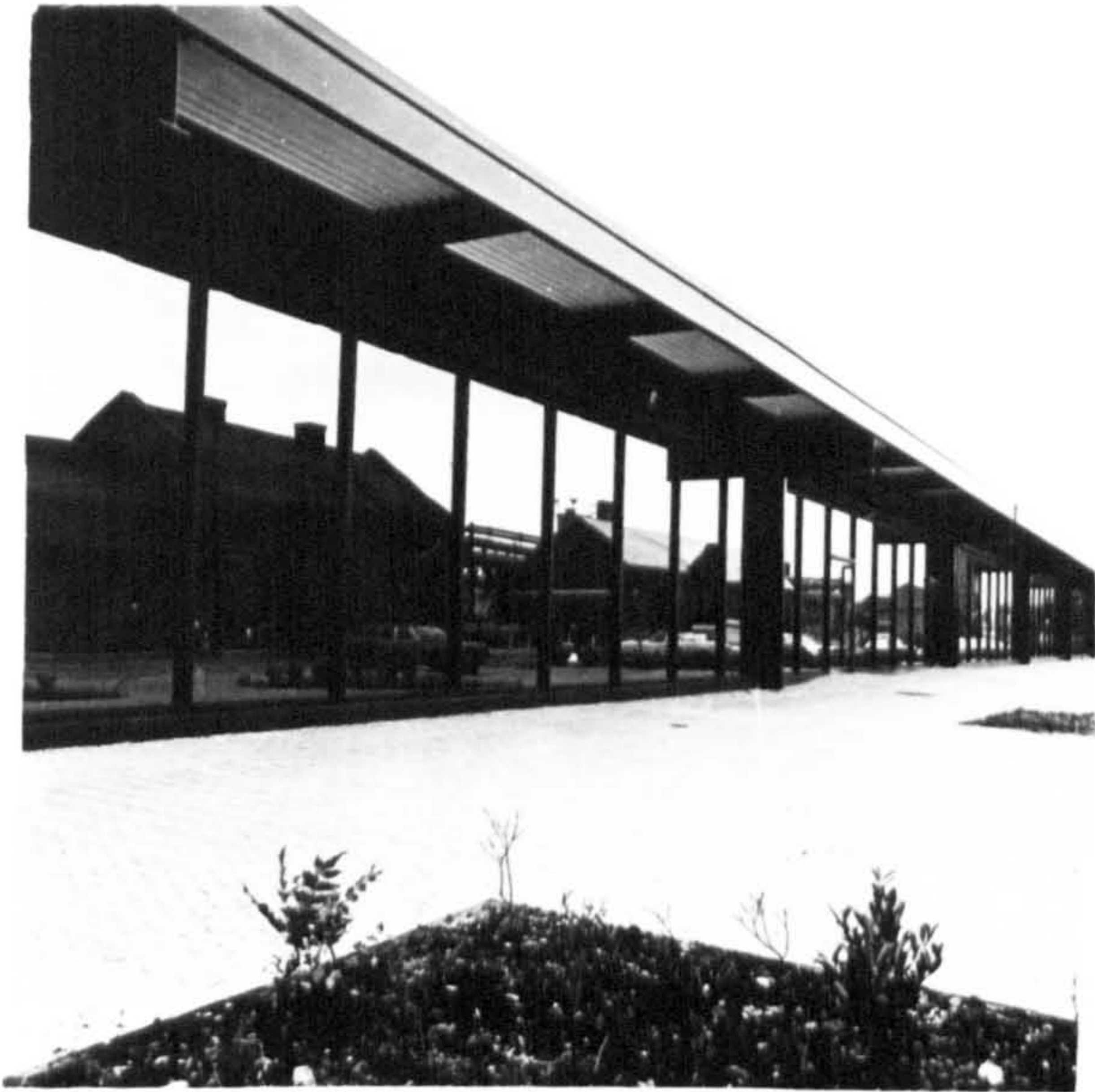
15. Aylestone Road Service Centre, Leicester, East Midlands Gas.
