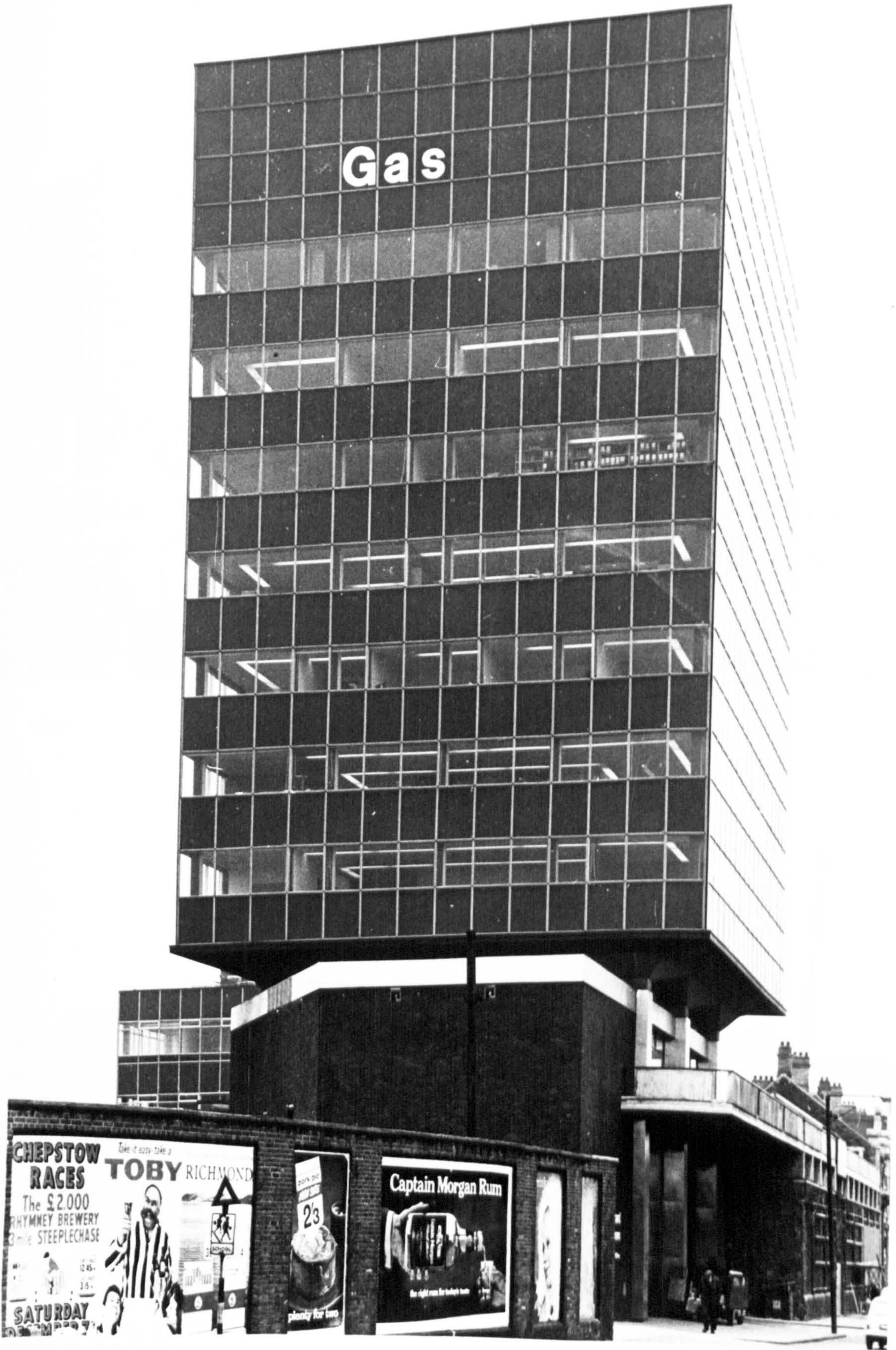
1. Snelling House, Cardiff, Wales Gas Headquarters.
