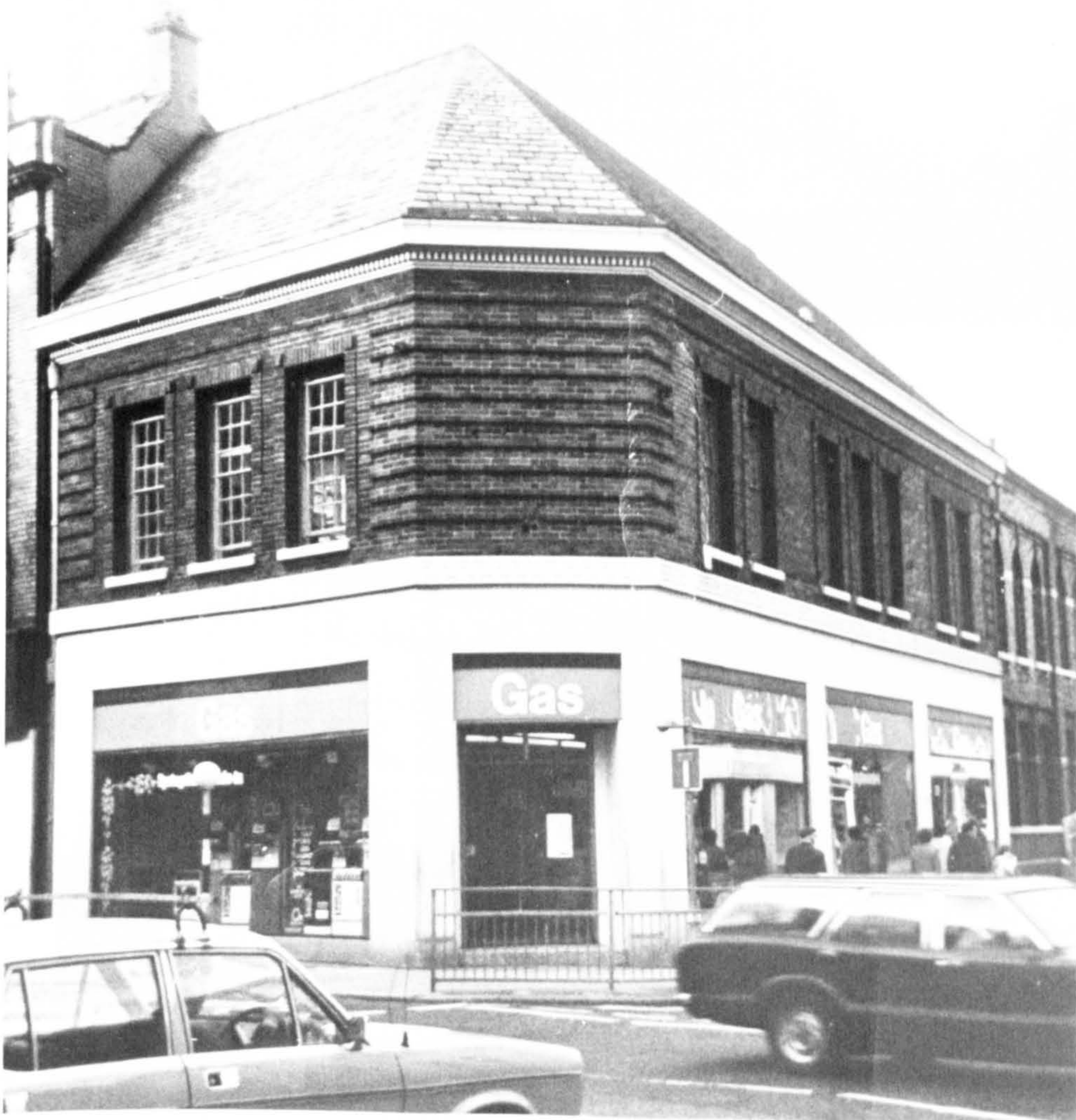
11. Altrincham Showroom, North West Gas.
