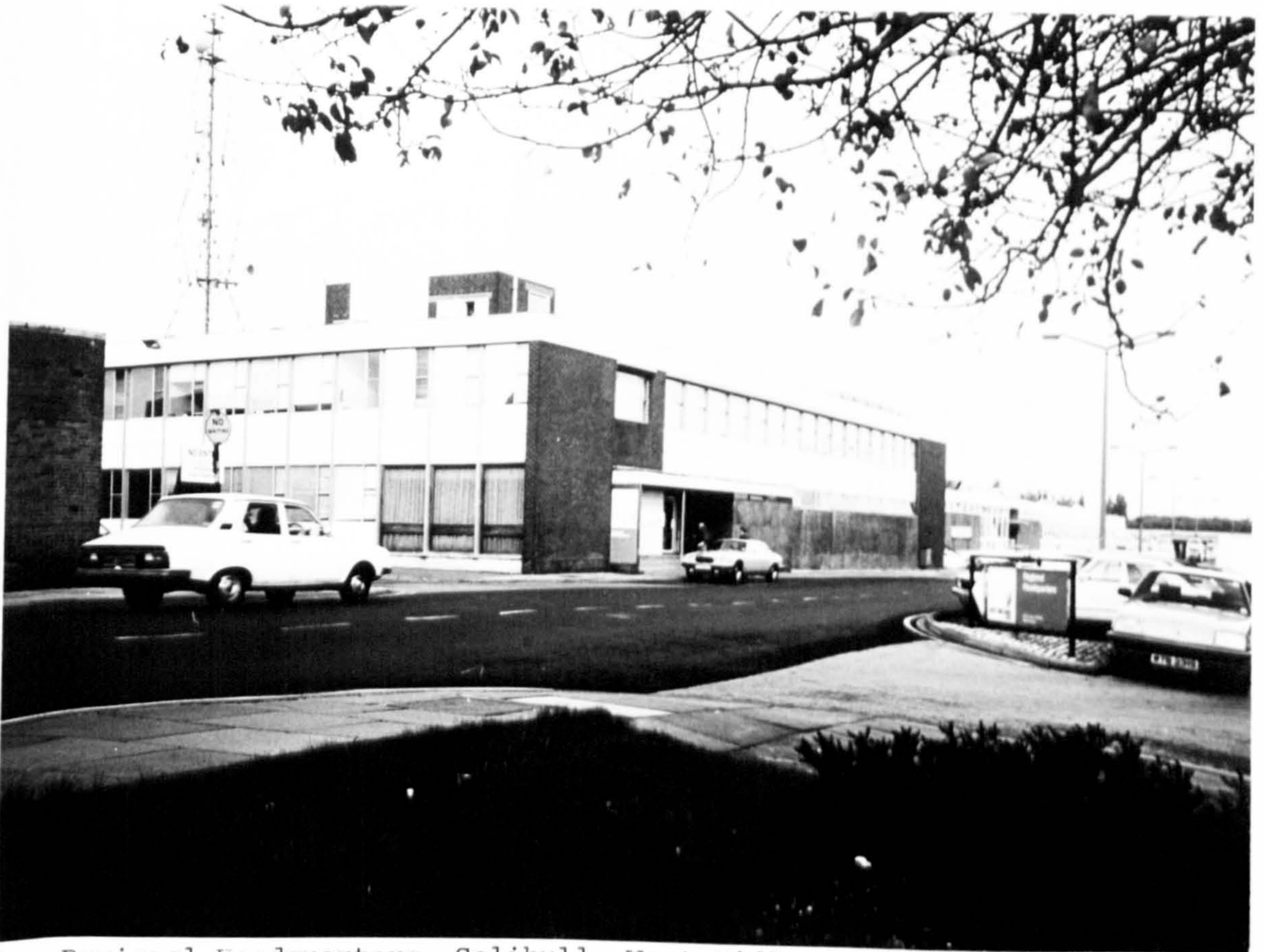
9. Regional Headquarters, Solihull, West Midlands Gas.
