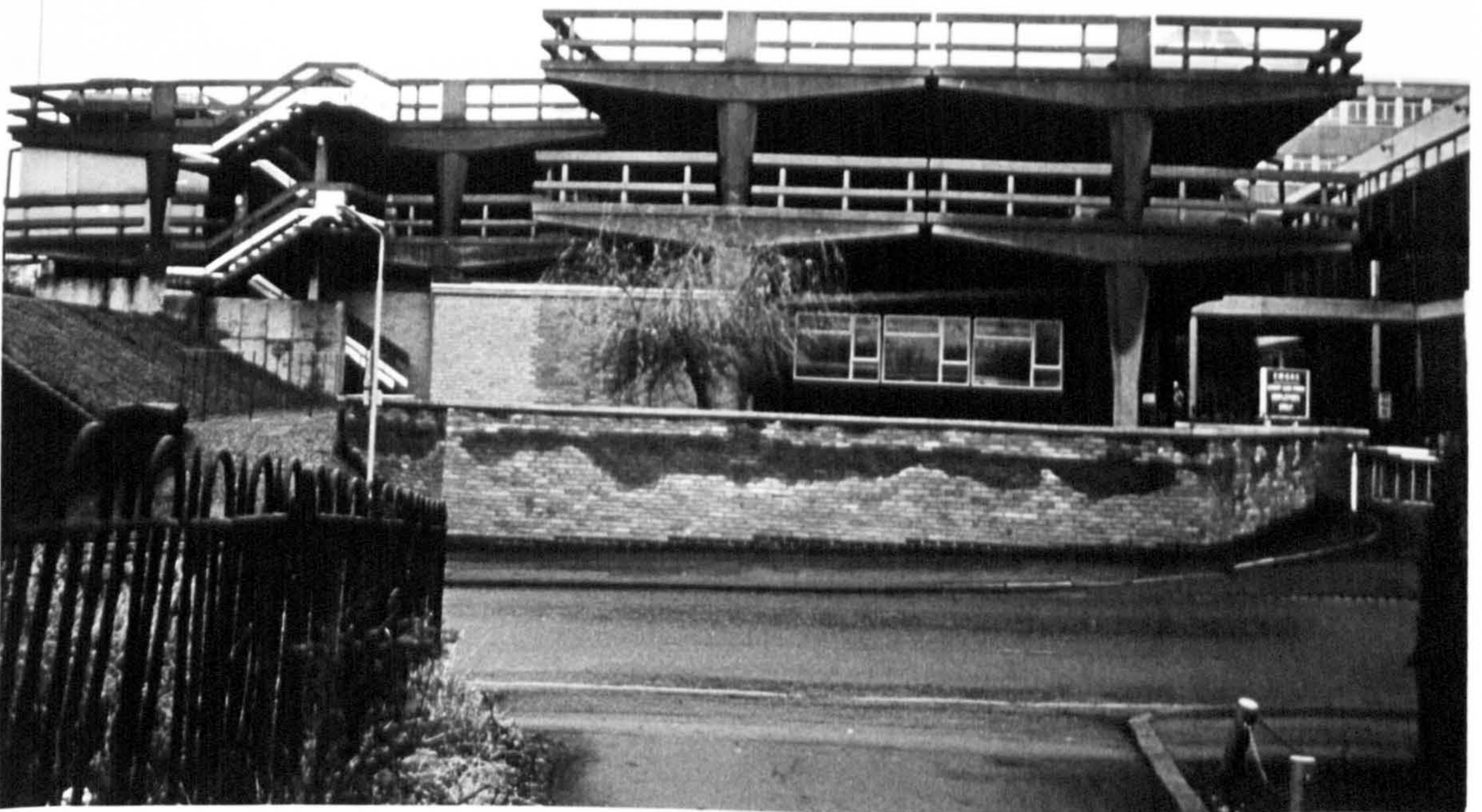
26. Car Parking Facilities, Regional Headquarters, Leicester, East Midlands Gas.
