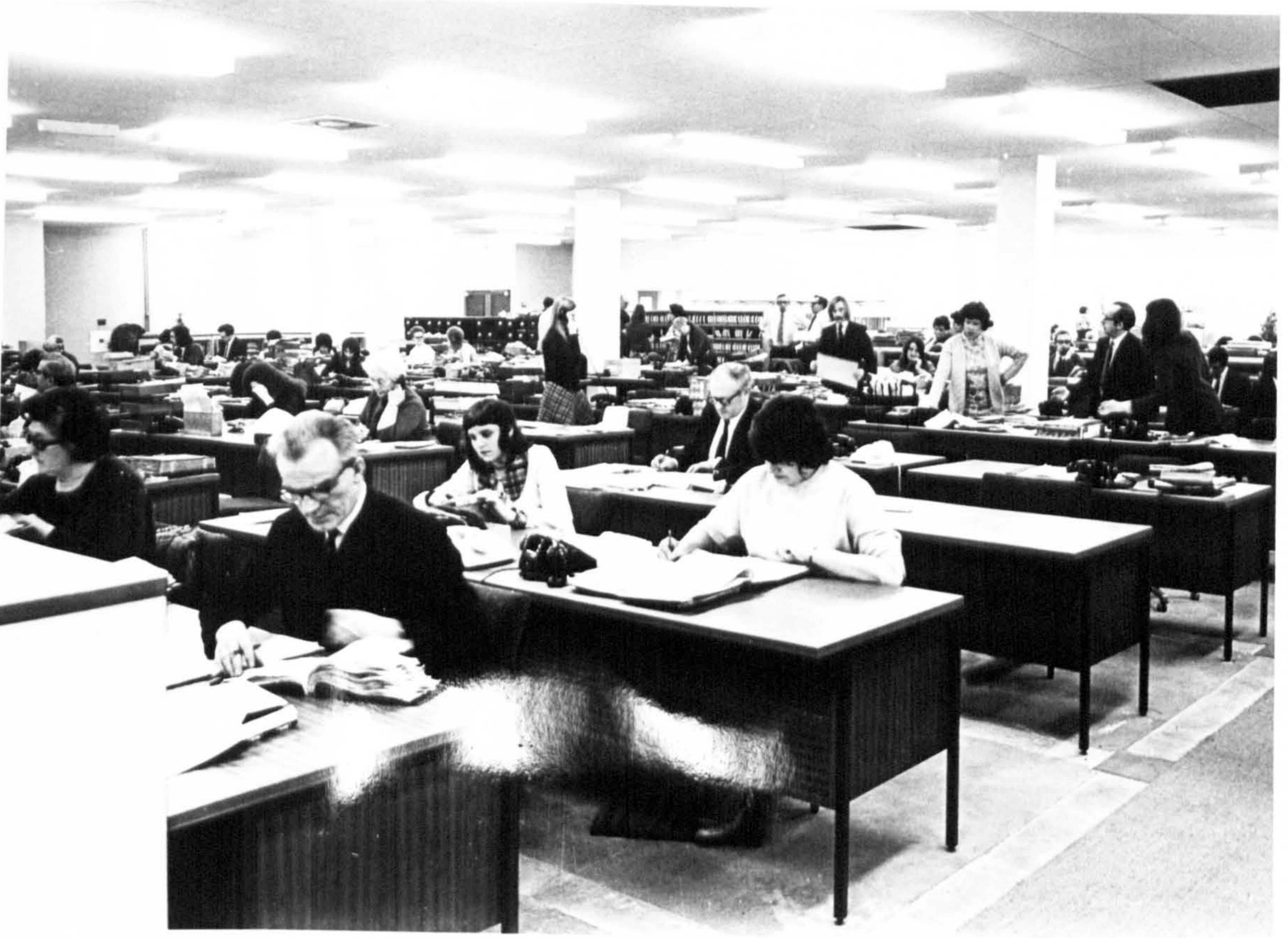
6. Interior, South Area Office, Wales Gas.
