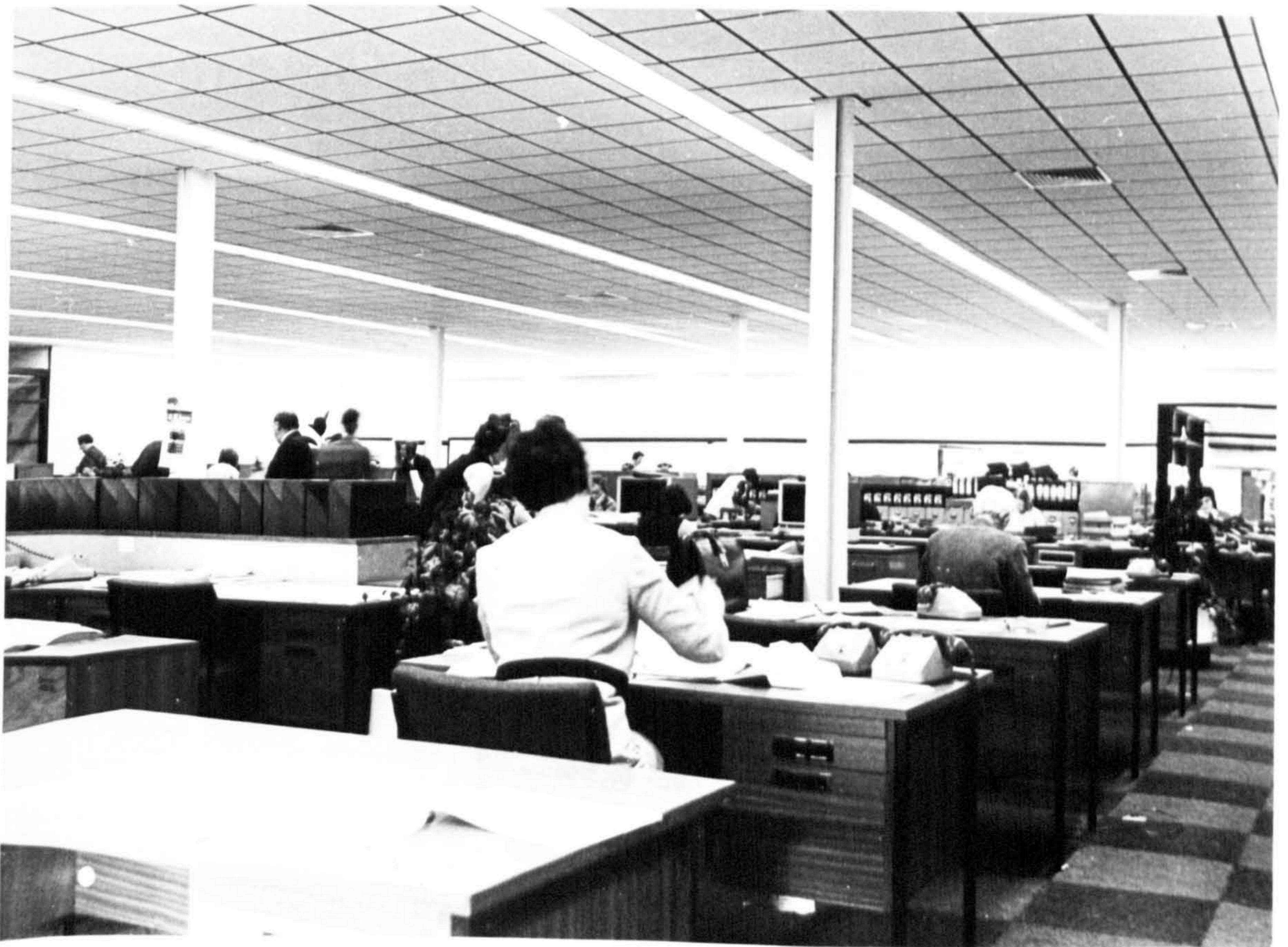
7. Interior, West Area Office, Wales Gas.
