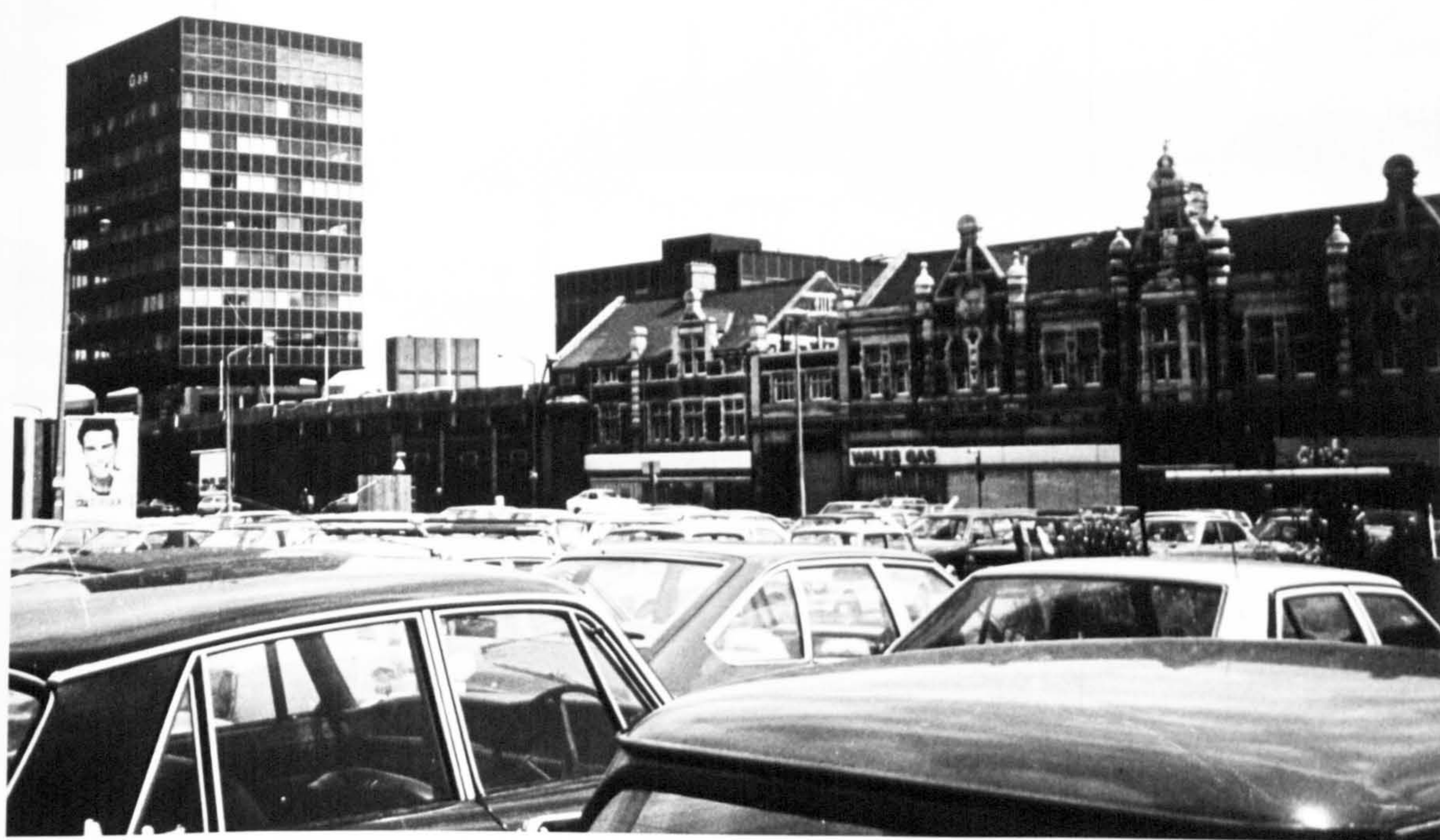
2. Snelling House and Bute Terrace, Cardiff, Wales Gas Headquarters.
