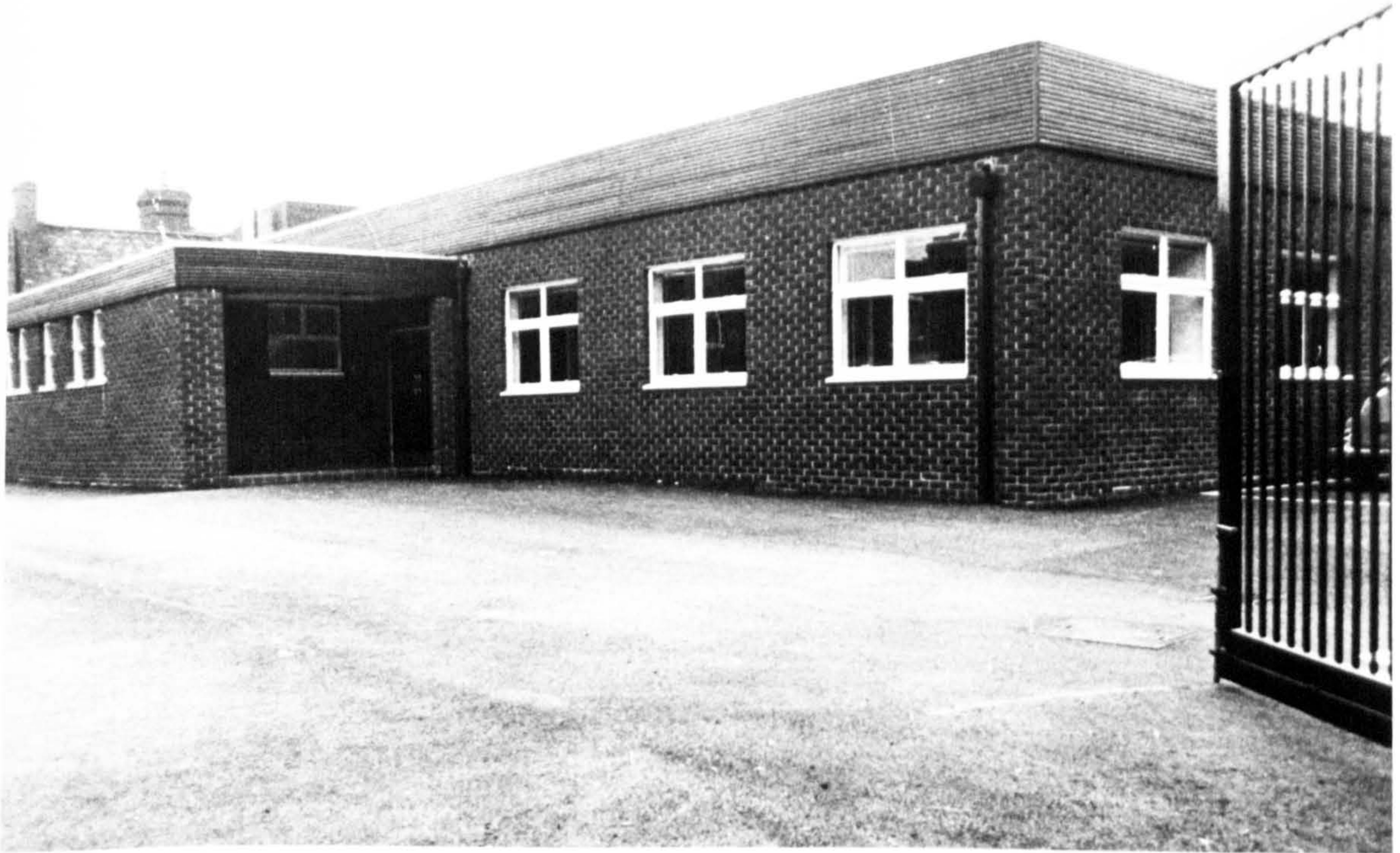
10. Nottingham East Depot, Great Freeman Street, Nottingham, East Midlands Gas.
