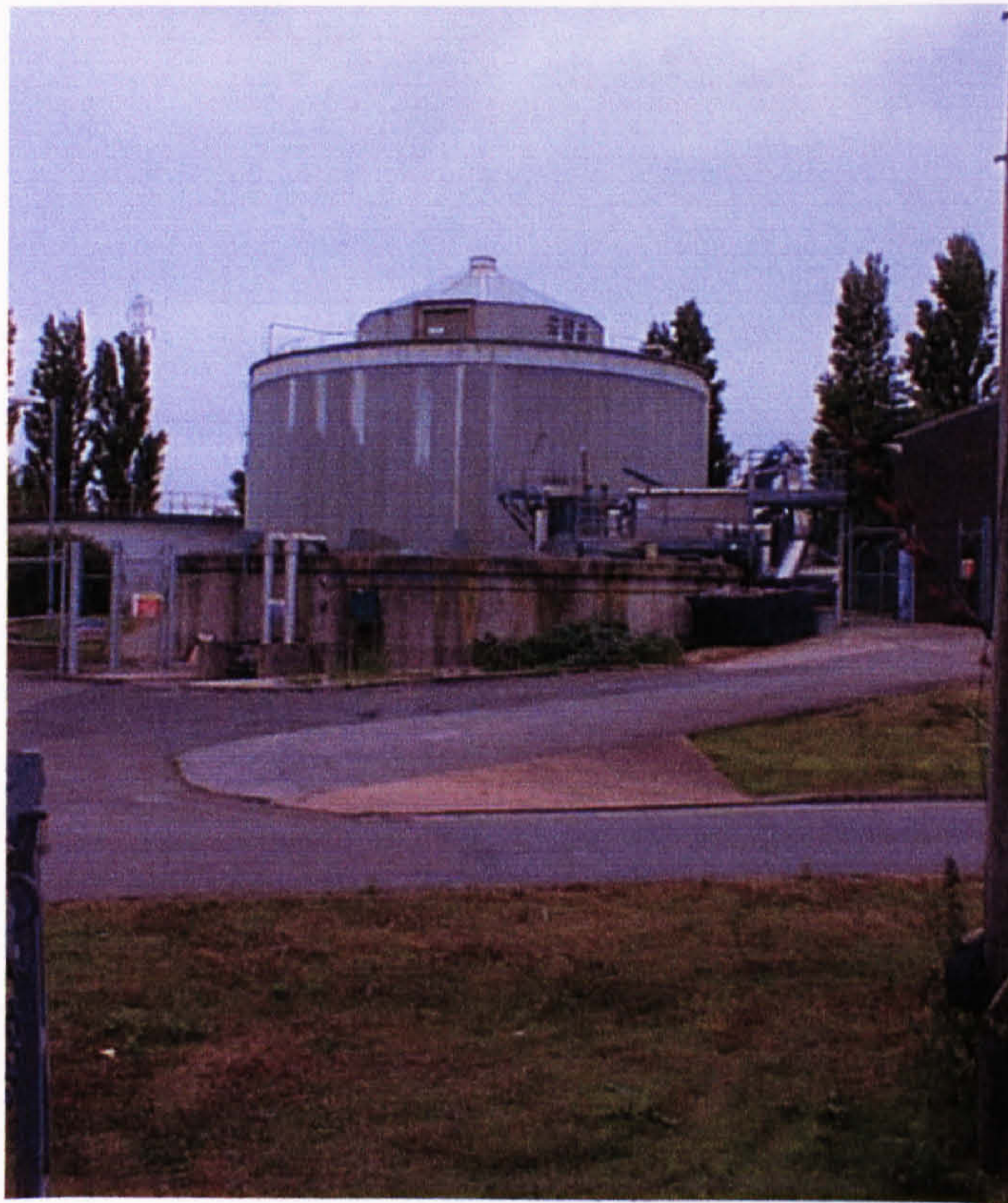
Figure 3.2. Mesophilic anaerobic digester at the Exeter treatment plant from which digesting sludge was obtained.
