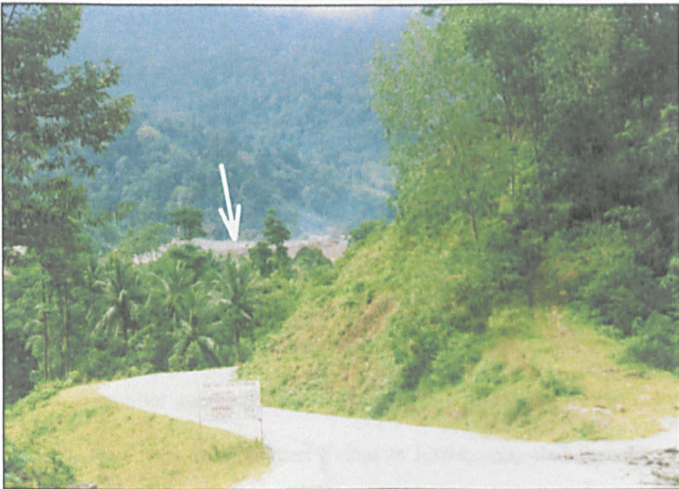
Fig. 4.1.2 At the edge of Lawar The road leading to the main construction site for the Pergau Dam (white arrow) which was clearly visible from the village.
