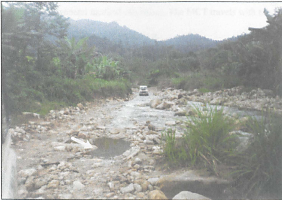
Fig. 4.4.4 The road to Rual. For a few hundred metres this stream forms part of the road. The Landrover has just left the soil track. This picture was taken in the dry season. The rest of the stream runs to the left from the point the Landrover entered the stream. Thousands of pools (see arrow) exist along the stream which contain clean water and are exposed to sunlight, providing ideal breeding sites for An. maculatus .
