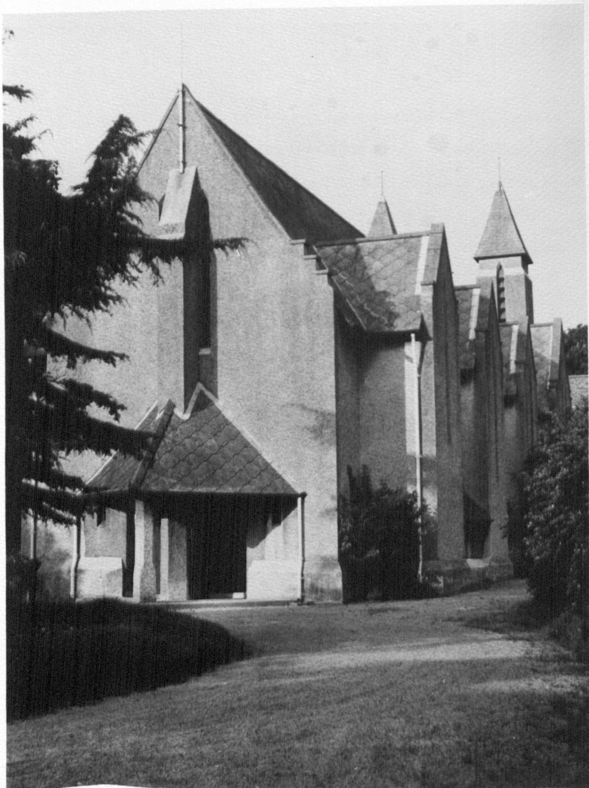
Plate 11. St. Winifred's Chapel from the south-west. It has roughcast walls and red asbestos cement tiles. Three transept gables have single lancets, the far one a pair. All are coped. The ambulatory roof can just be seen. The turrets are shouldered. The severity of the design gives no anticipation of the rich interior. The photograph was taken after the second world war, when the tree in the turning space, left, had had time to grow. It was planted at the time of the consecration.
