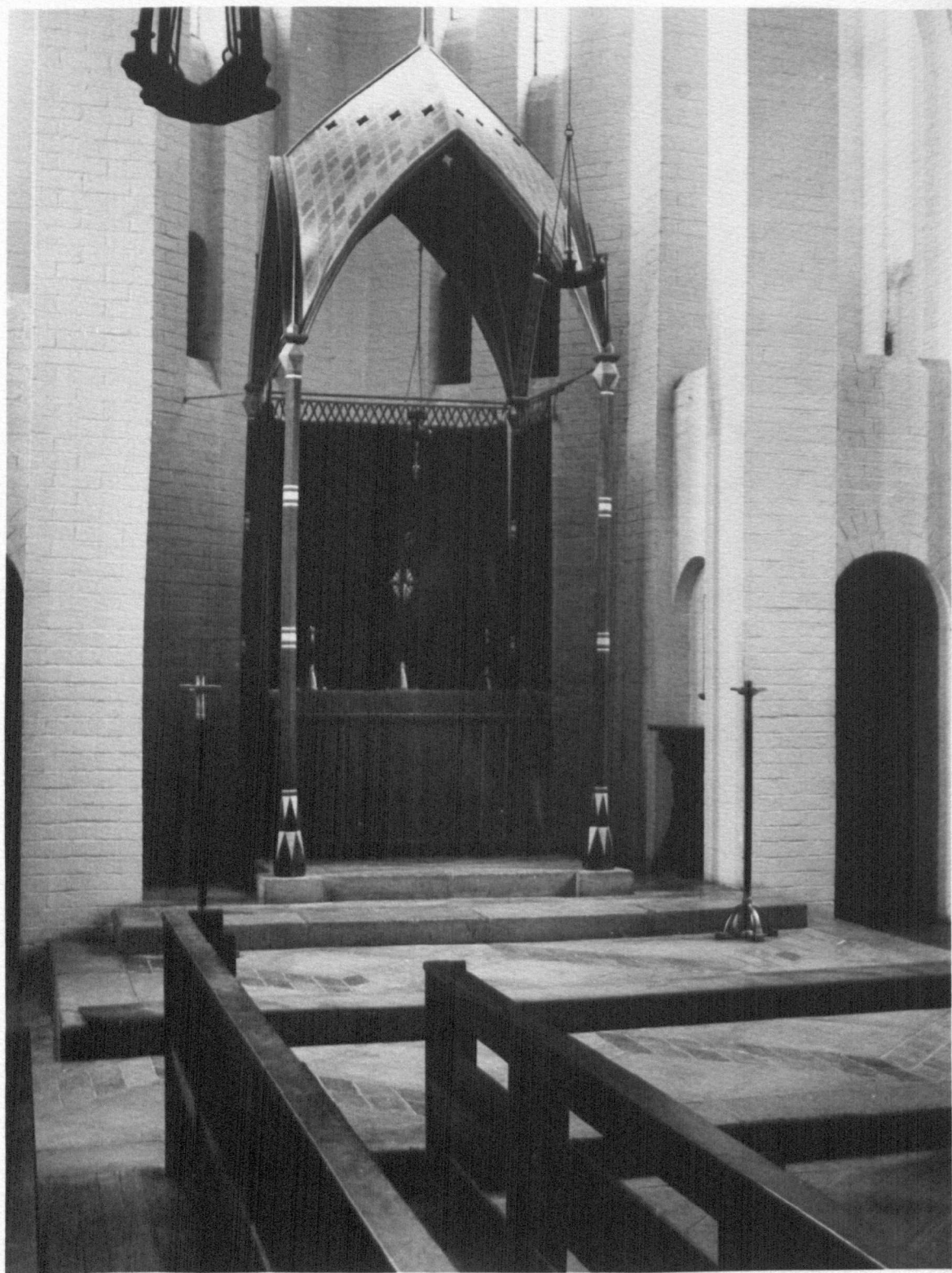
Plate 7. The altar and its ciborium, with the openings from the music wing behind. The canopy was trellised in red and blue, and encircled by perforations. The finial is out of the picture. The paving was concrete. The stalls were of walnut.
