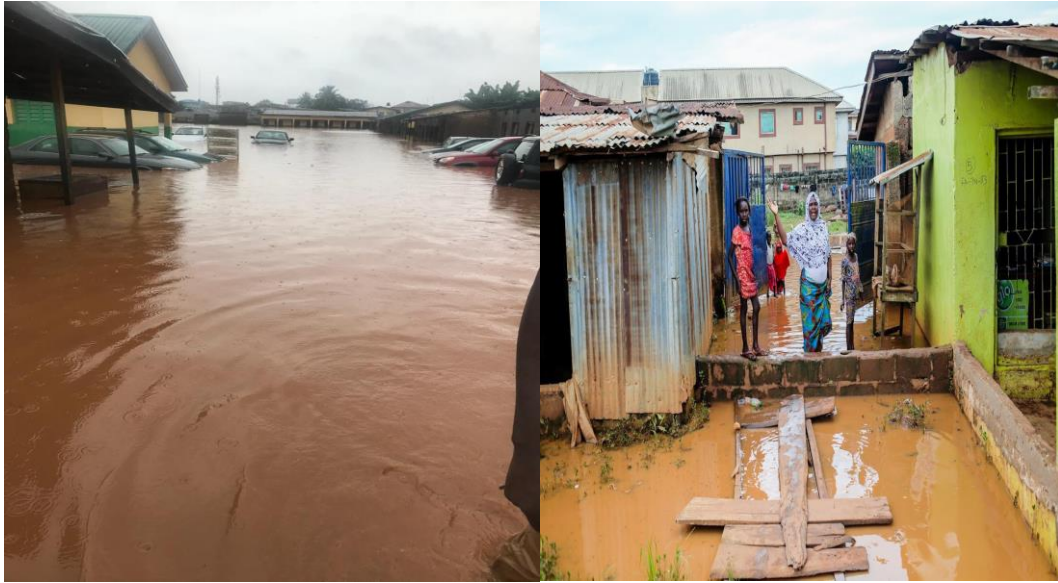
Figure 1.2: a) Flooded school; b) shops flooded following heavy rainfall in Ijebu-Ode.
