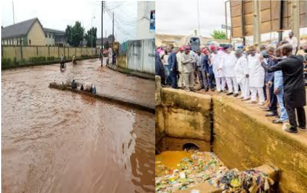
Figure 1. 8: a) & b) flooded streets/roads and narrow and blocked drainage in Ijebu-Ode.
