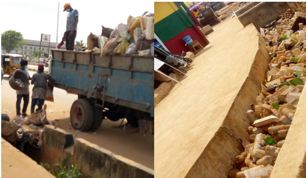
Figure 1.5: a) poor waste collection; b) excessive rubbish in the drain in Ijebu-Ode.
