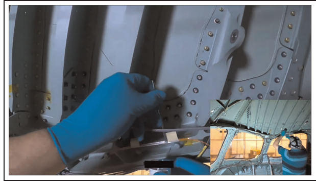
Figure 4. Installation of sensors in a fuselage test. Main image is a view from operator headset, inset figure shows a wide view of the installation area.
