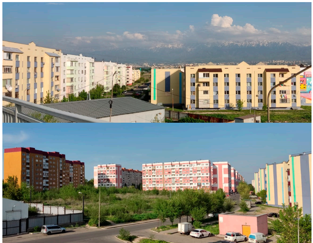
Figure 2. Views of the surveyed social housing complex, Almaty, Kazakhstan.
