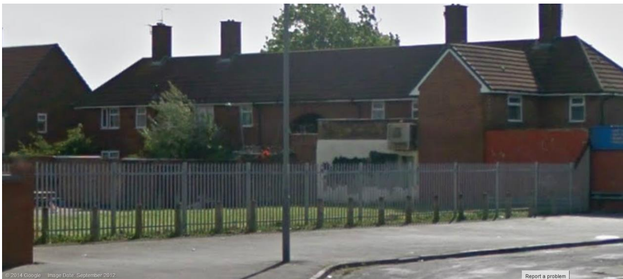
Figure 8: Fenced off, the same site in September, 2012. Image provided by Google Street Maps.
