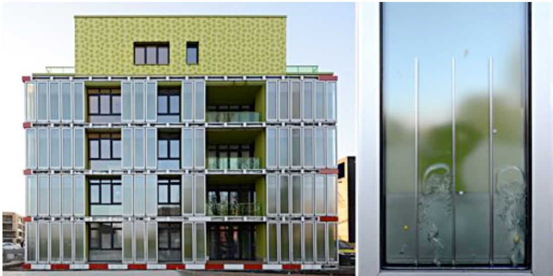
Figure 9: Photobioreactor façade by Splitterwerk and Arup, Hamburg, Germany. Images copyright Arup Deutschland GmbH, Colt International GmbH and SSC GmbH.
