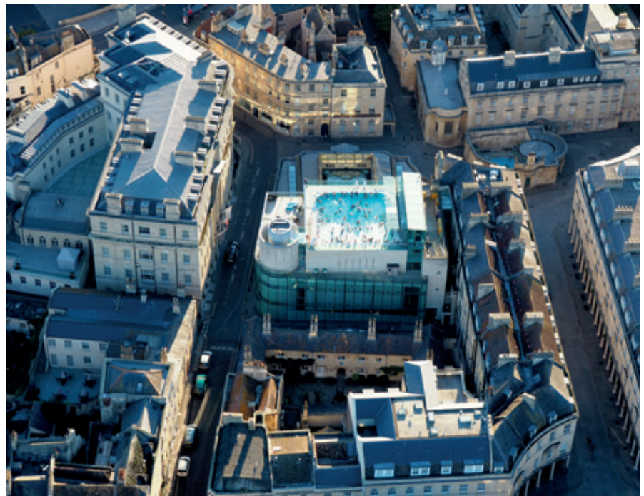
Nicholas Grimshaw's roof-top baths of limestone and glass, slotted neatly into the Georgian townscape of Bath alongside the conserved and regenerated Cross Bath, top right (Photo: Jonathan Taylor)
