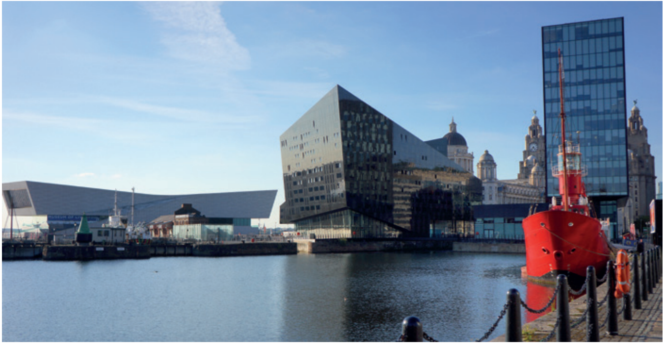
Regeneration on Liverpool's waterfront: the long low sweep of 3XN's Museum of Liverpool to the left, and Broadway Malyan's glossy black wedge-shaped Latitude Building in the centre: the two towers of the Royal Liver Building and the dome of the Port of Liverpool Building can be seen behind the tall office block at 1 Mann Island to the right (Photo: Peter de Figueiredo)
