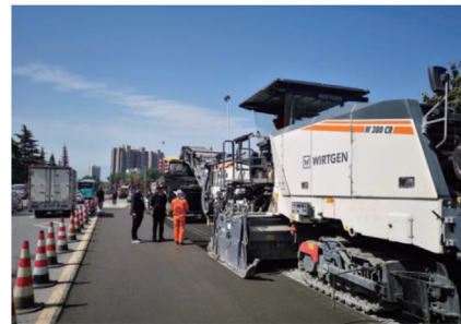
Fig. 78. Construction site of W380CR foam asphalt cold in-situ recycling unit. (a) Homogeneous foamed bitumen cold recycling mixture. (b) Intelligent and efficient regeneration.
