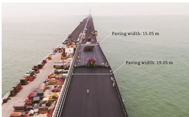
Fig. 71. Continuous widening paving of Hong Kong–Zhuhai–Macao Bridge.
