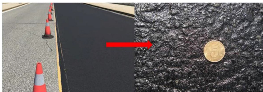
Fig. 39. Field application of fog seal technology (Xu et al., 2022a).
