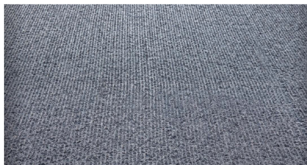
Fig. 76. Pavement texture after fine milling.
