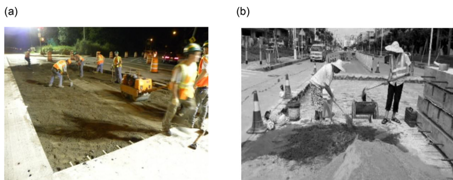
Fig. 57. Prefabricated pavement base layer. (a) Sand cushion course (Tayabji, 2016). (b) Dry-mixed mortar (Tang, 2019).
